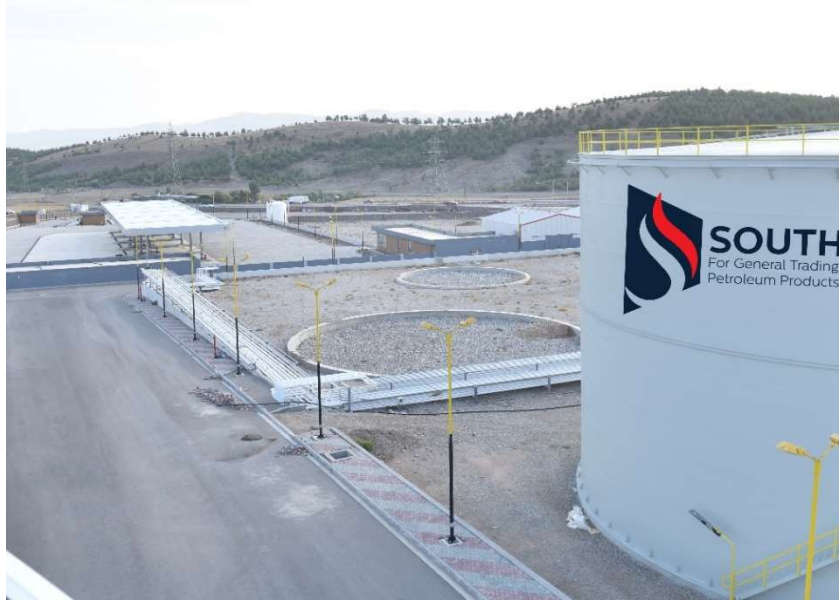
Concrete ring wall foundation
